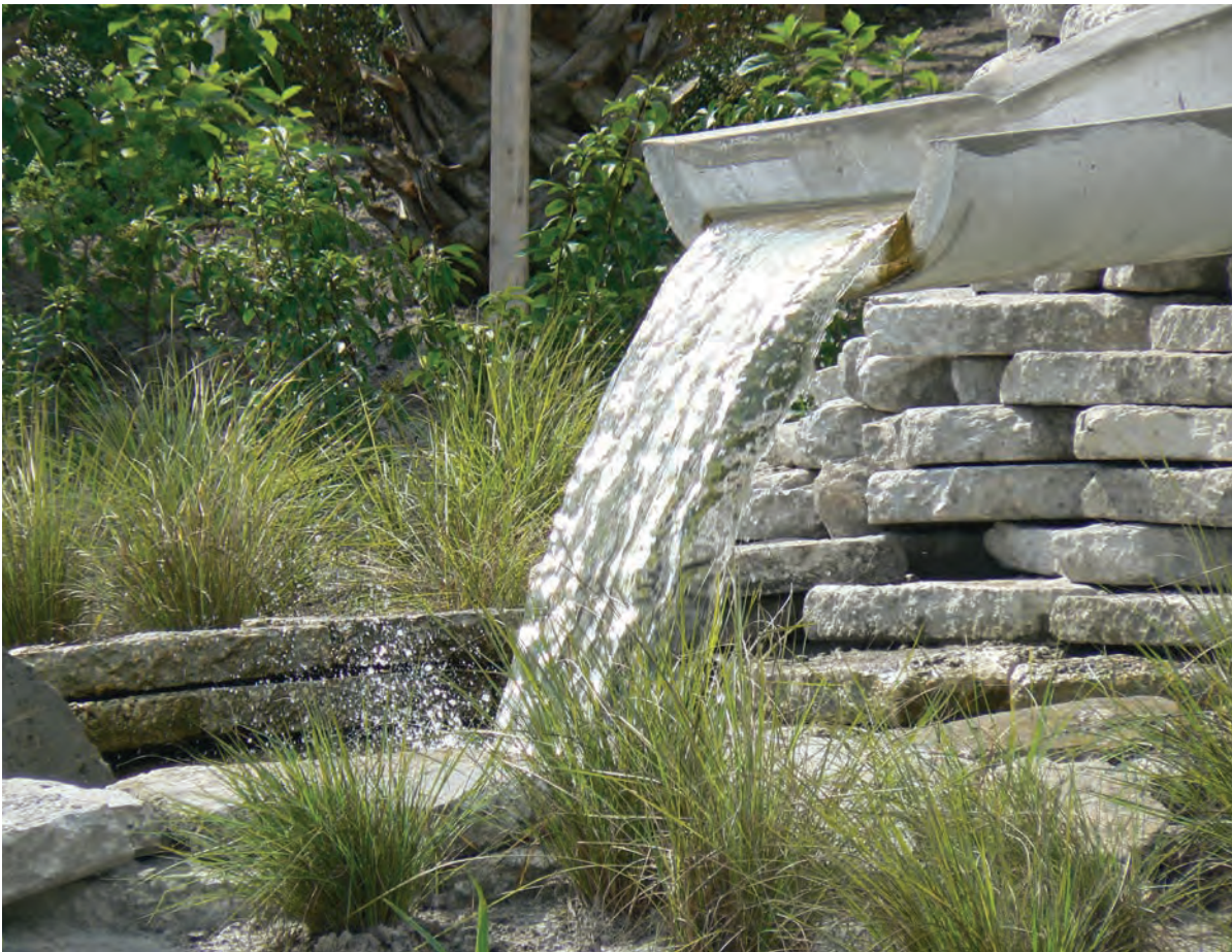
◀ Lucy Keshavarz's eco-art project Babbling Brook in Palm Beach County, Florida, uses a cut stormwater pipe for the fountain and recycled sidewalk slab as the retaining wall and edging for the brook that circulates the stormwater. Photo by Lucy Keshavarz
