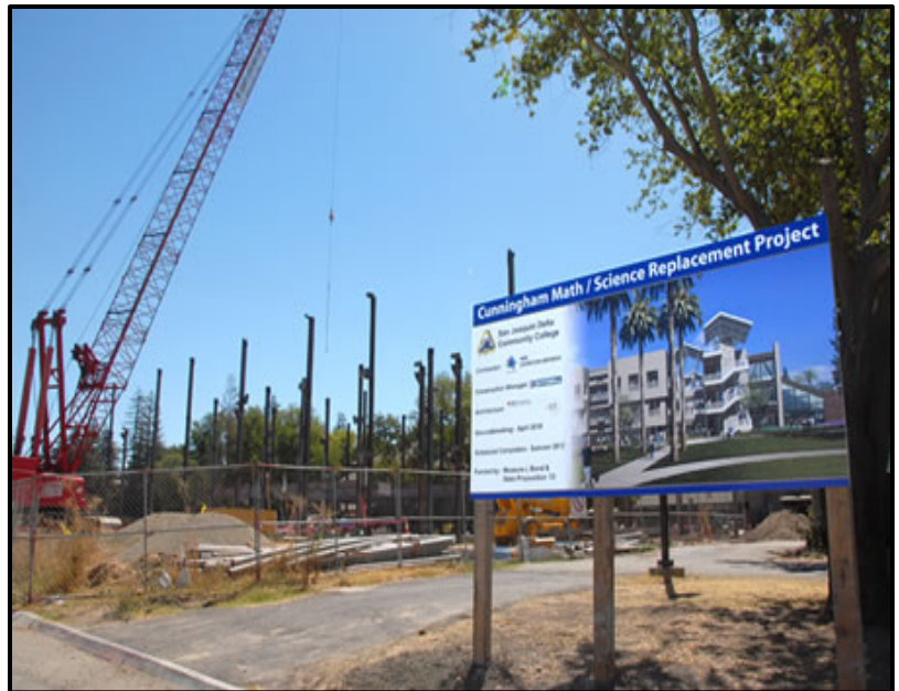
Construction of Delta's New Science and Mathematics Building
