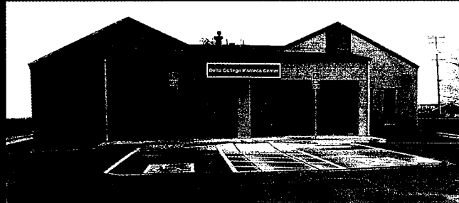
Existing Classroom Building
