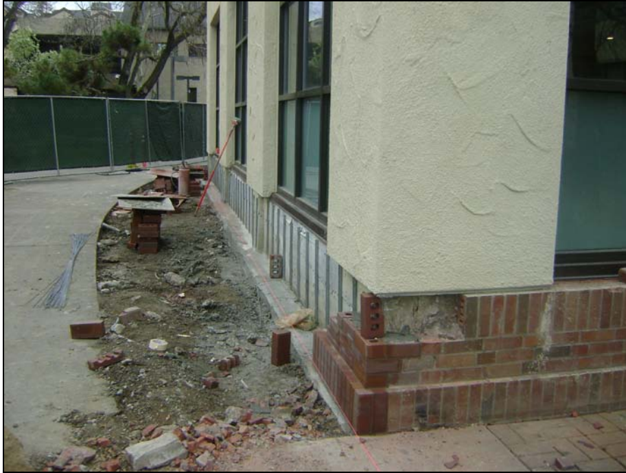
The exterior brick work begins
