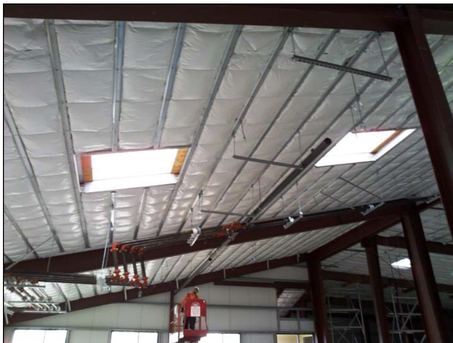
Overhead Utility Rough-in – Hydronic Piping
