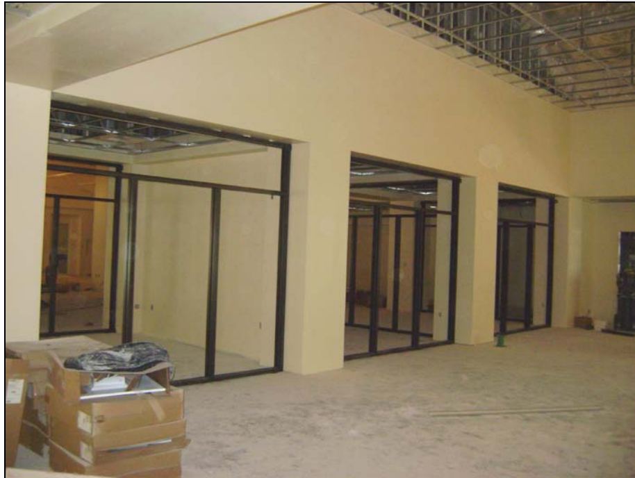
Installation of Interior Storefront Glazing continued
