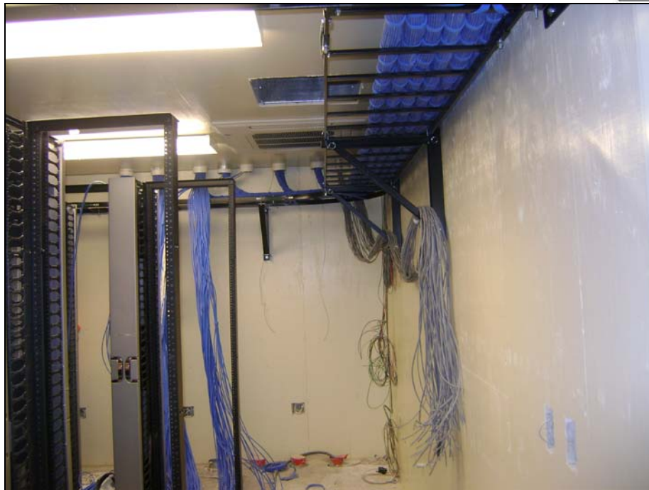
Data Cable installation continued at the Telecom Rooms
