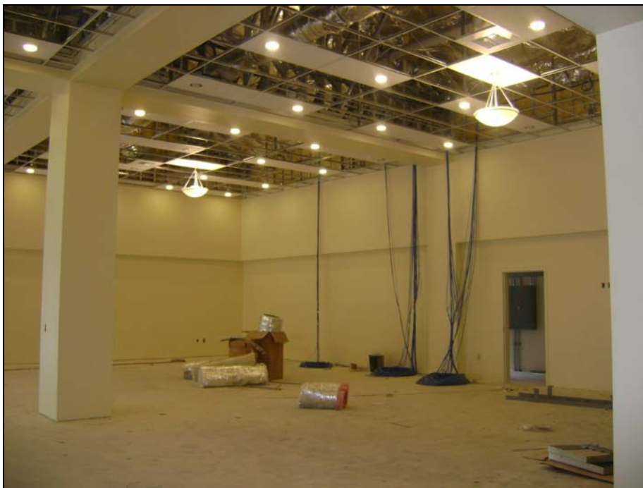
Light Fixtures were installed in the 2 nd Floor T-bar
