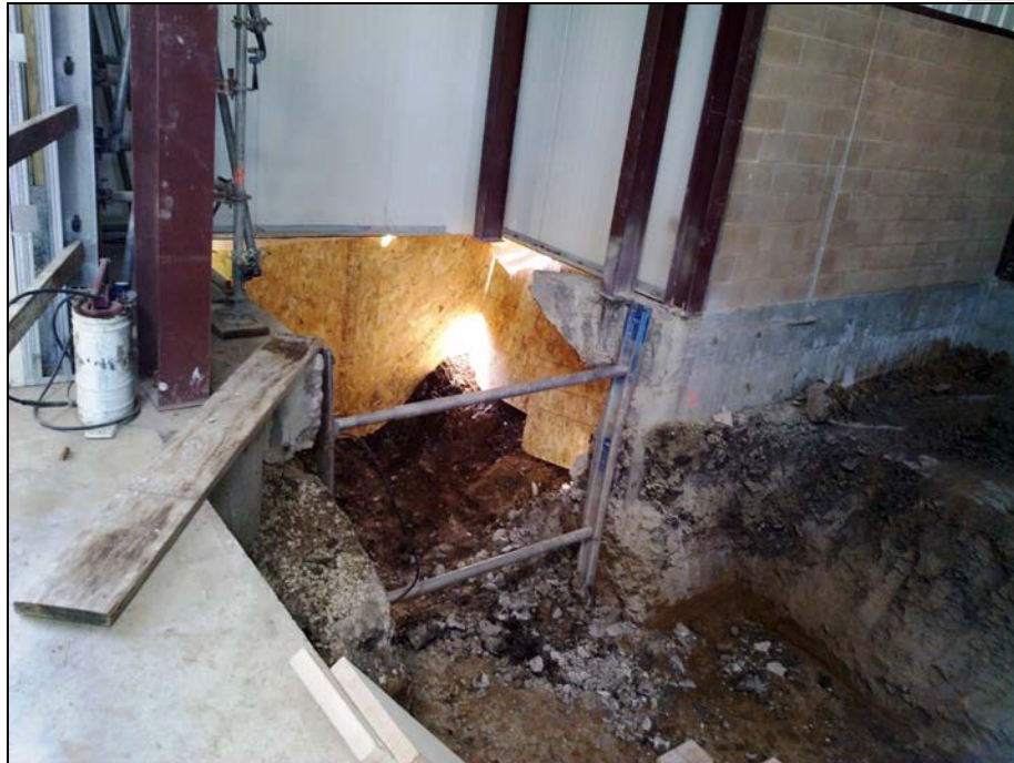
Foundation Demolition for Duct Trench
