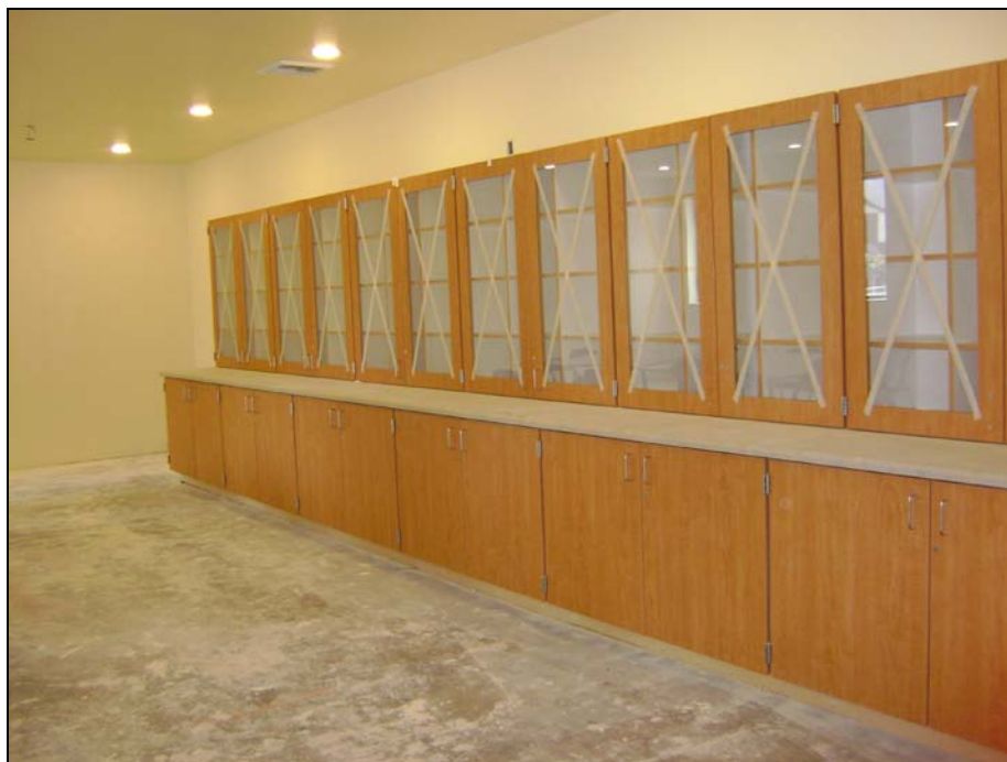
Casework installation continued
