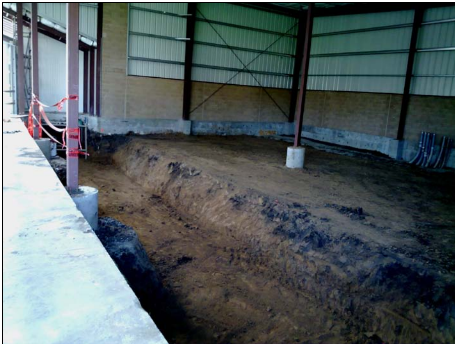
HVAC Duct Trench Excavation
