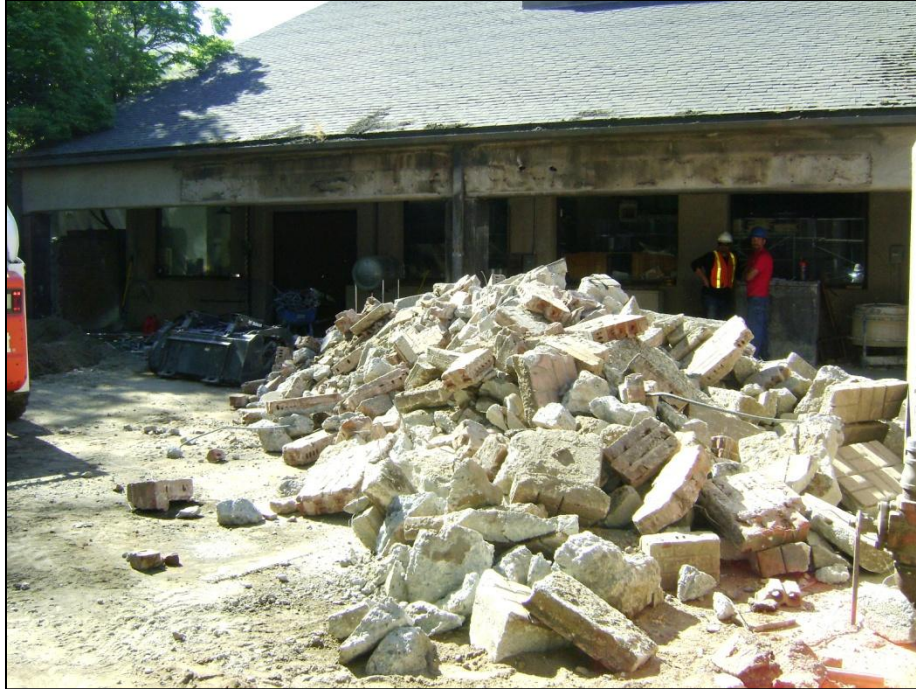
Shima Art Yard – Demolition Activities
