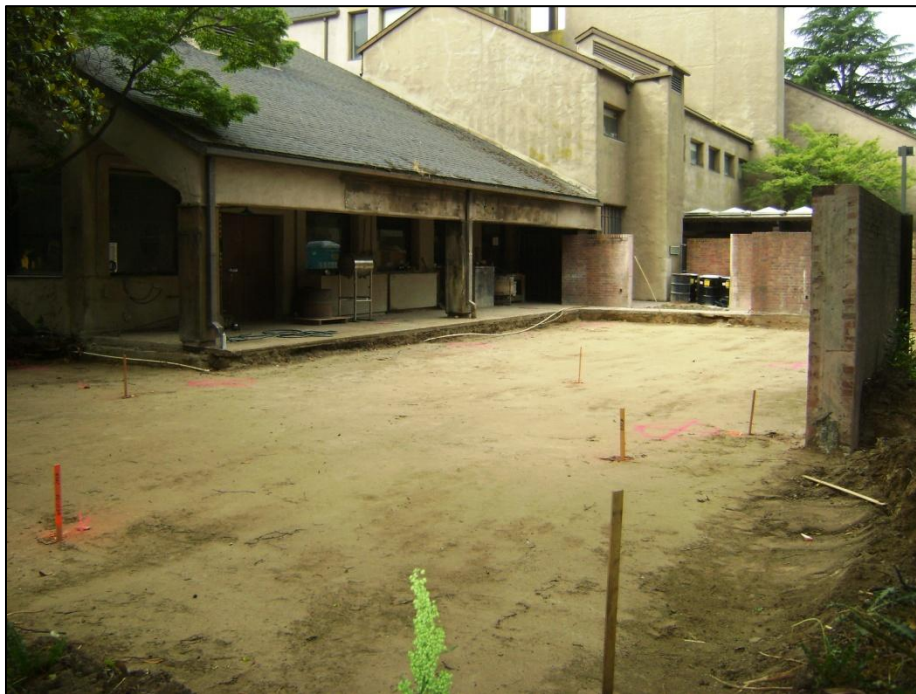
Shima Art Yard – Rough Grade Established
