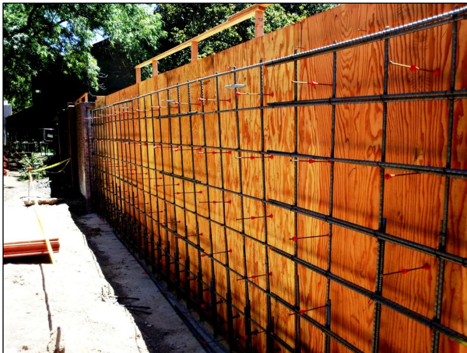
Shima Art Yard – Wall Formwork and Reinforcing
