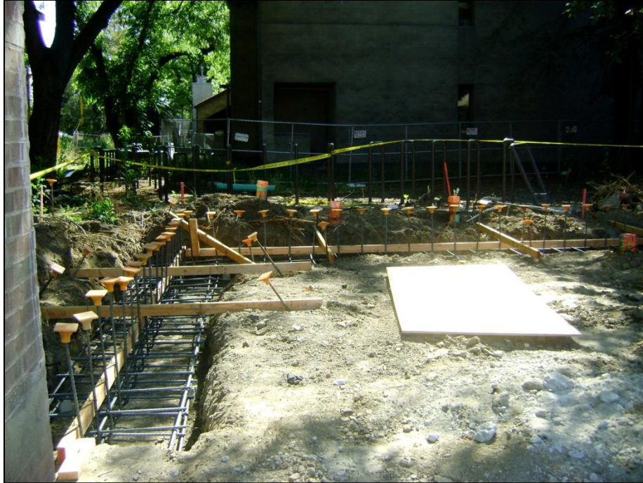
Shima Art Yard – Wall Footing and Reinforcement
