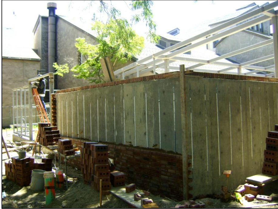
Shima Art Yard – Brick Veneer Installation
