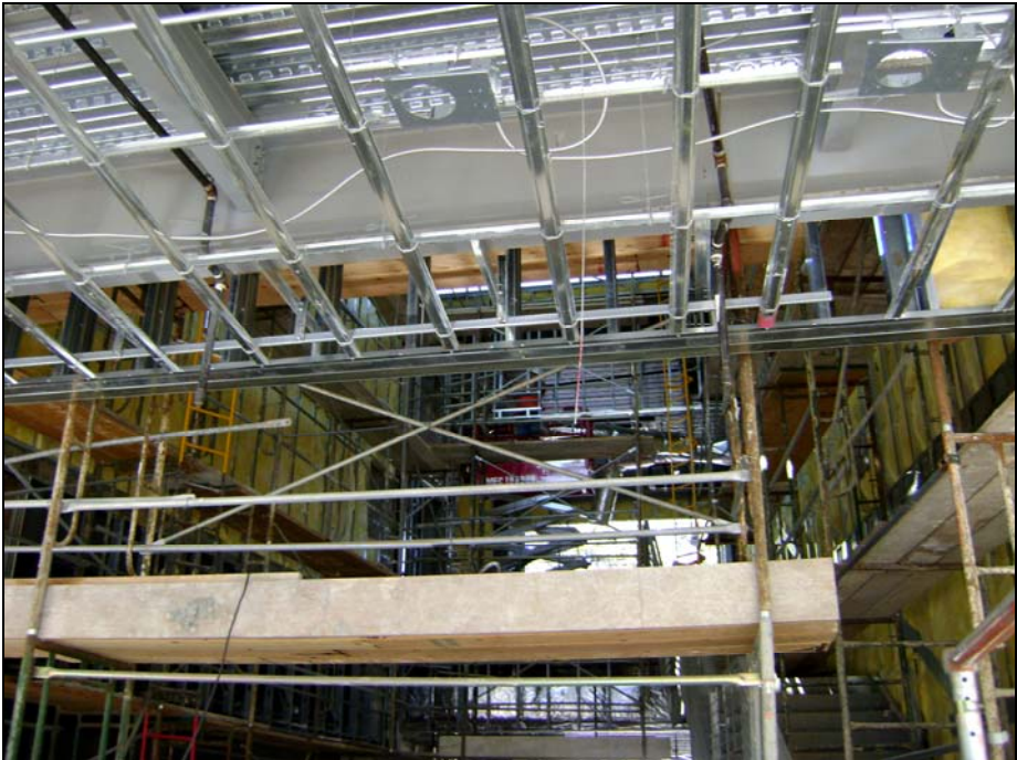
Interior Ceiling Framing
