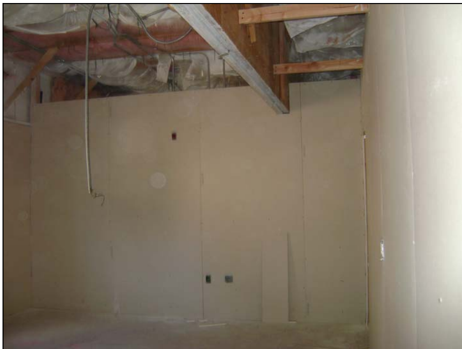
Sheetrock Installation
