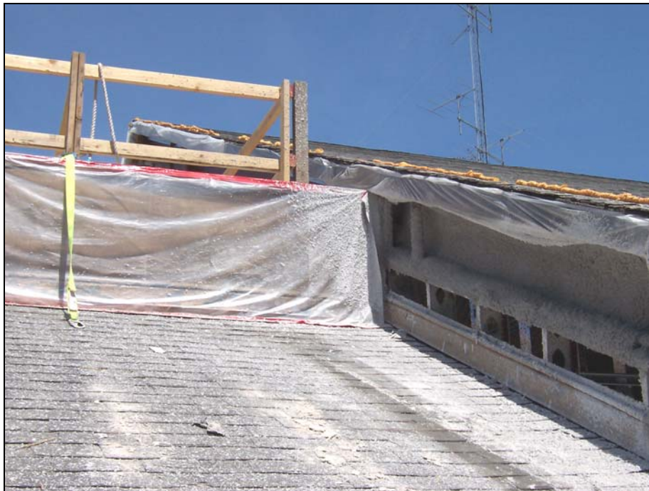
Fireproofing Installation @ Building Perimeter
