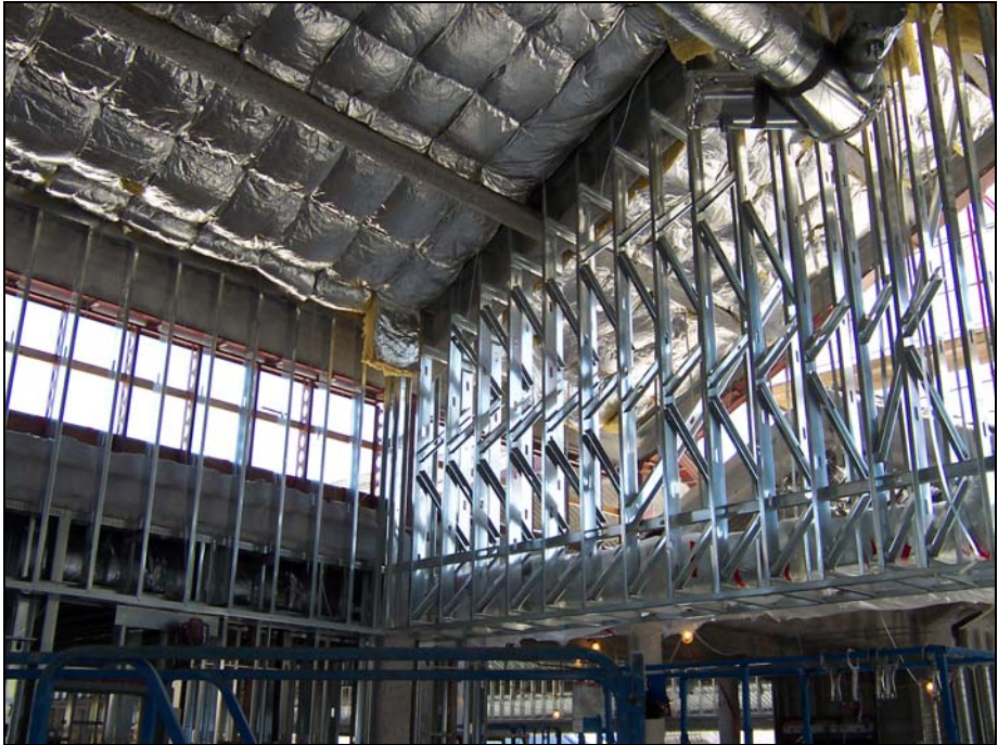
Interior Metal Stud Framing at Second Floor
