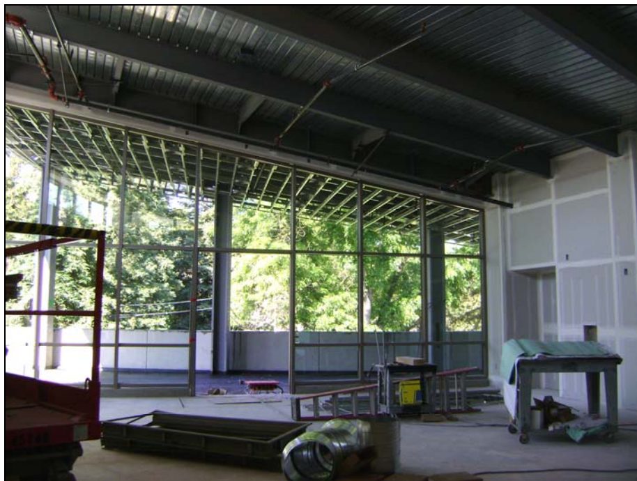
Storefront Window System South Side
