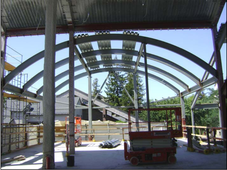
Installation of Structural Steel at Northeast Corner of Building
