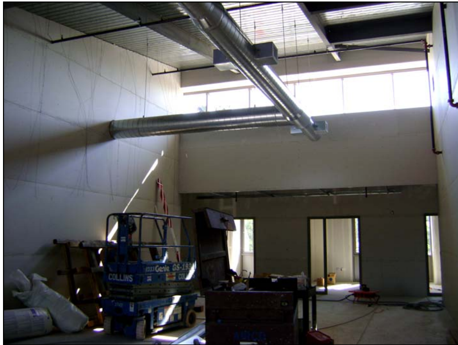
Interior Ductwork, Clearstory Windows, Drywall
