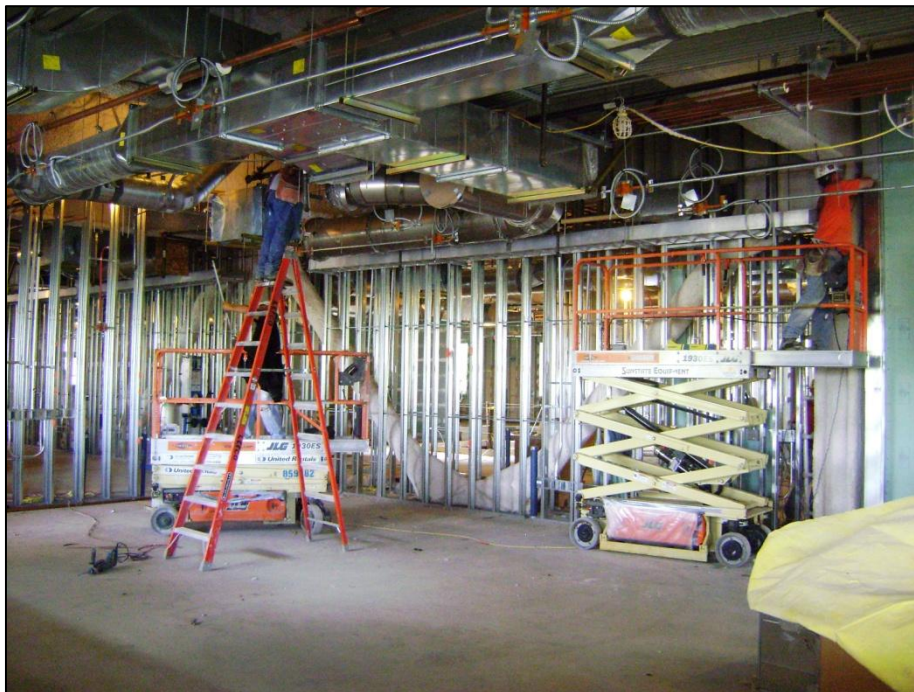
HVAC Duct Installation
