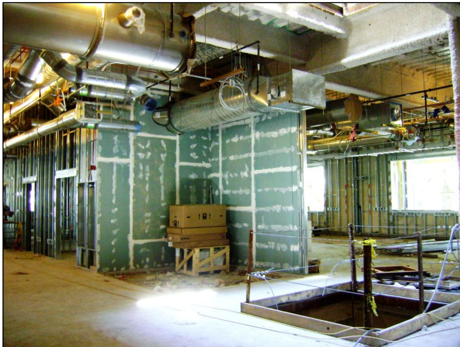
Building Wing A HVAC Shaft Wall Framing
