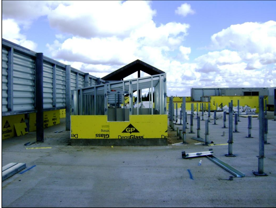
Building A Roof Framing and HVAC Duct Support Steel
