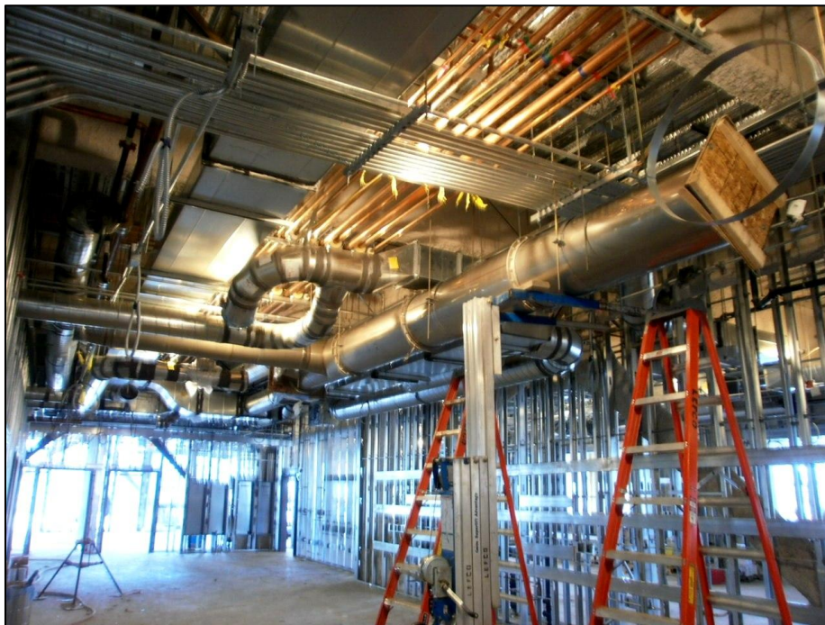
Stainless Steel HVAC Duct Installation
