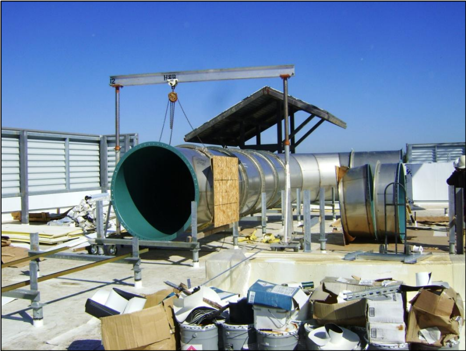
Building A - HVAC Duct Installation
