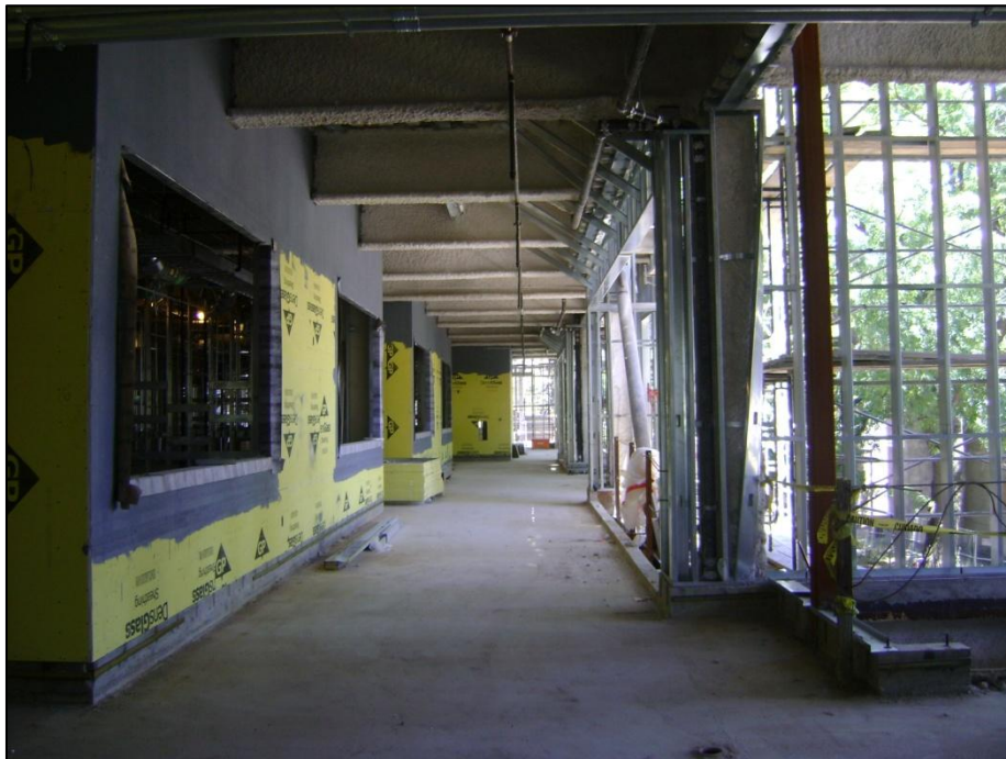
Building A – Second Floor Corridor
