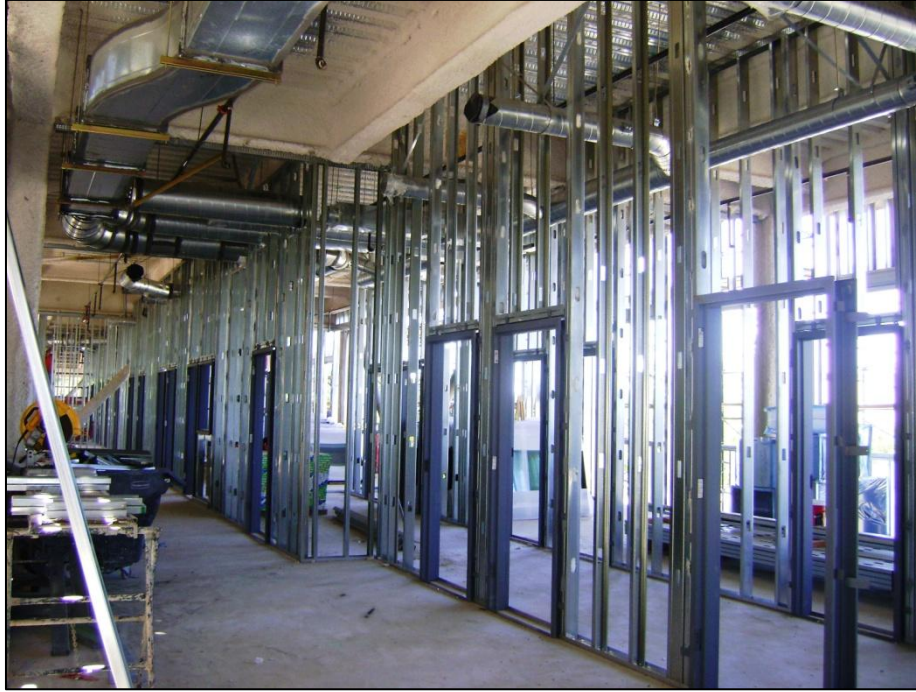
Building B – Interior Framing
