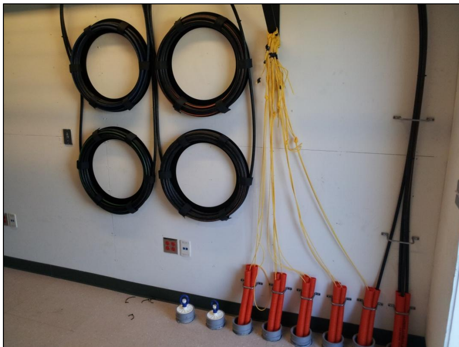
Data Center – Fiber Optic Cable Installation
