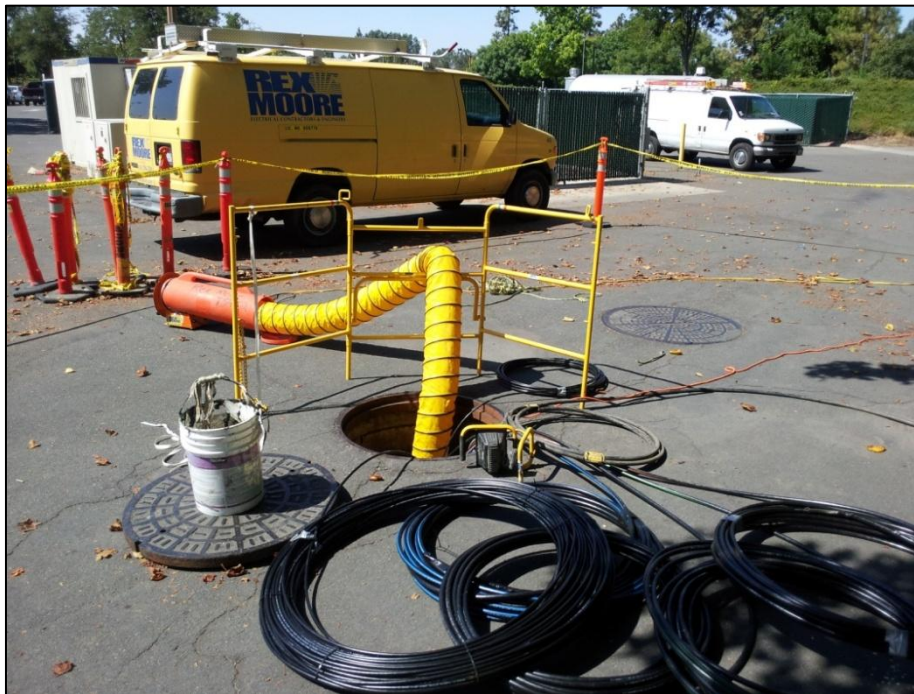
Fiber Optic Cable Installation in Process
