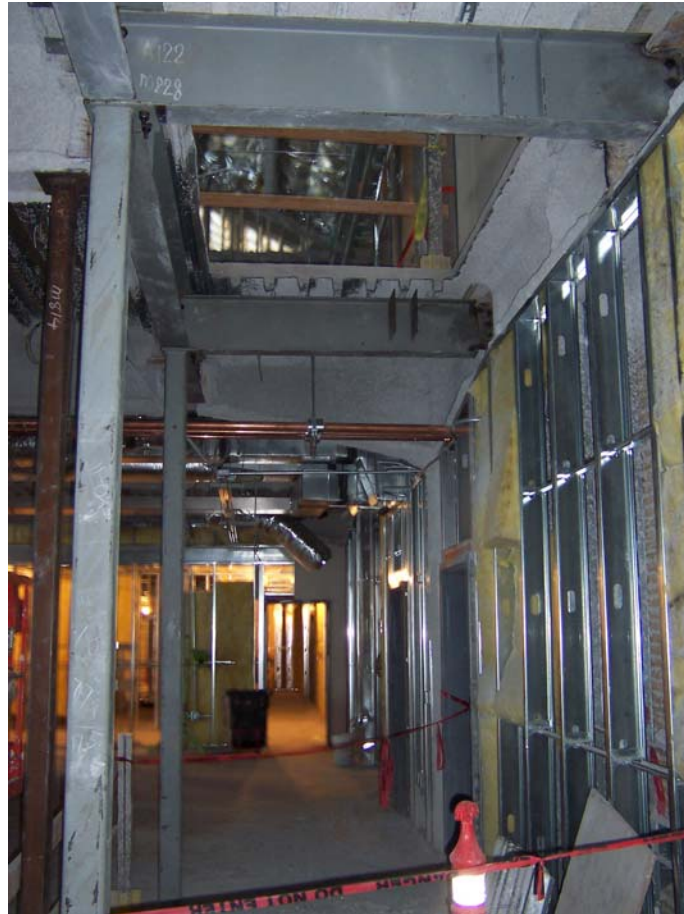
Structural Modifications at Southern Elevator
