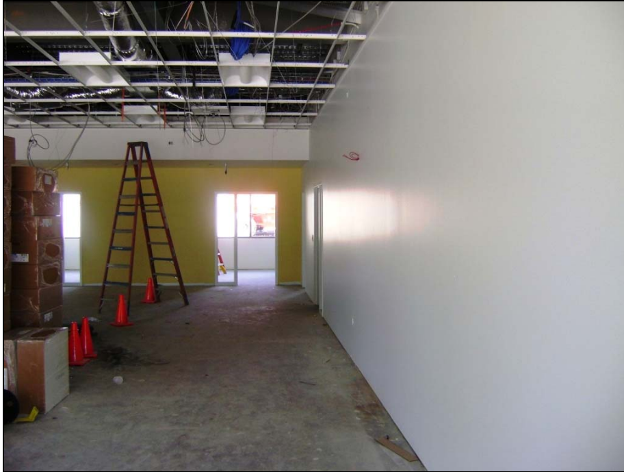
Interior Ceiling Framing, Light Fixtures and Finish Paint
