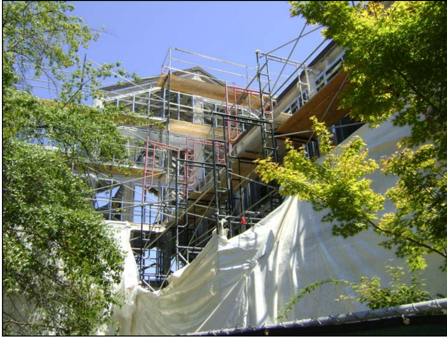
New Exterior Metal Framing
