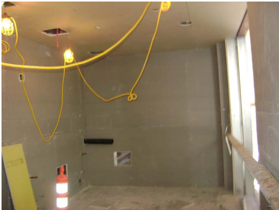
Installation of Interior Gypsum Wallboard
