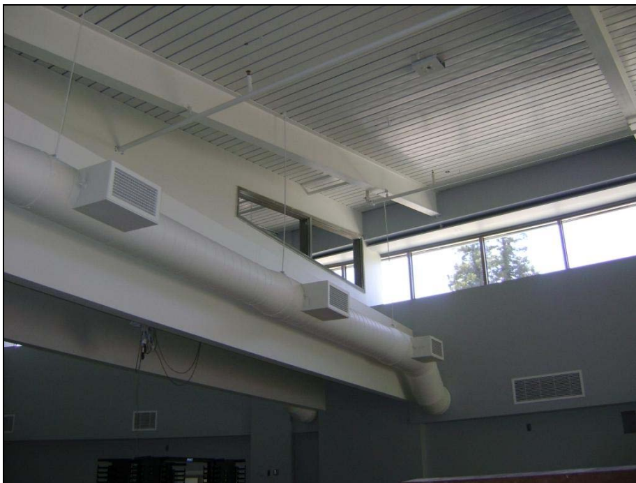
Finish Ductwork, Clearstory Windows and Paint
