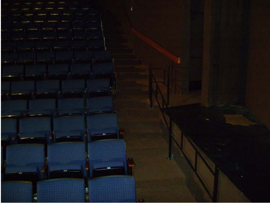
Tillie Lewis – Partial View of Handrail Installation in Progress
