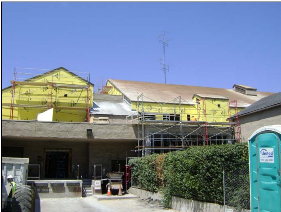
Installation of Exterior Gypsum Wallboard
