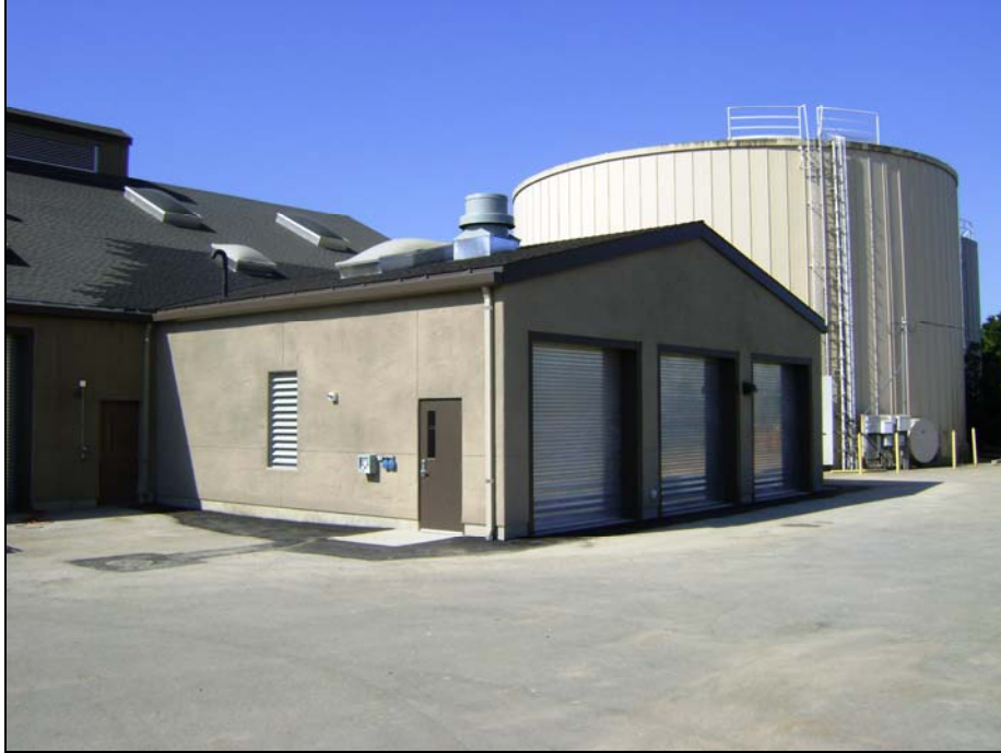
Chiller Building Addition
