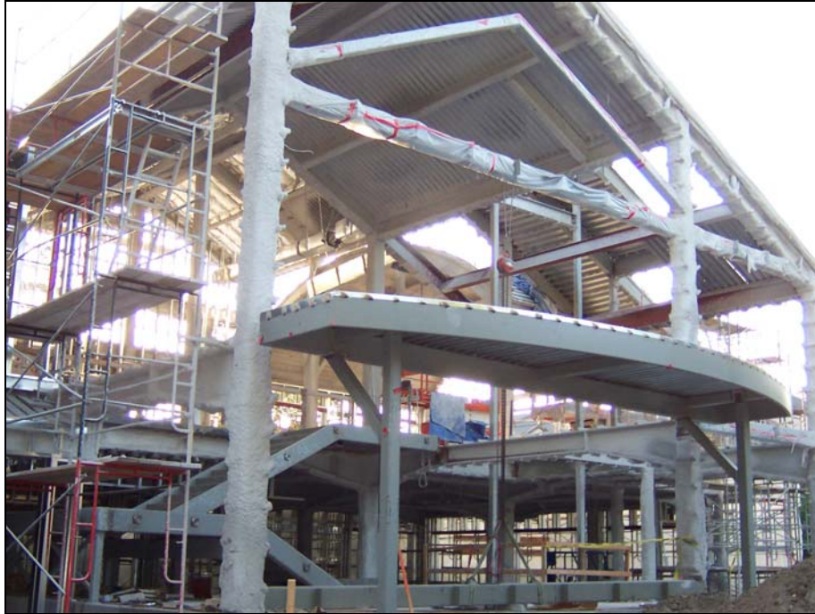
Improvements at Entry/Lobby
