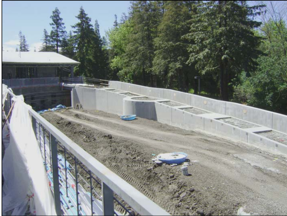
Retaining walls and ramp at West entrance
