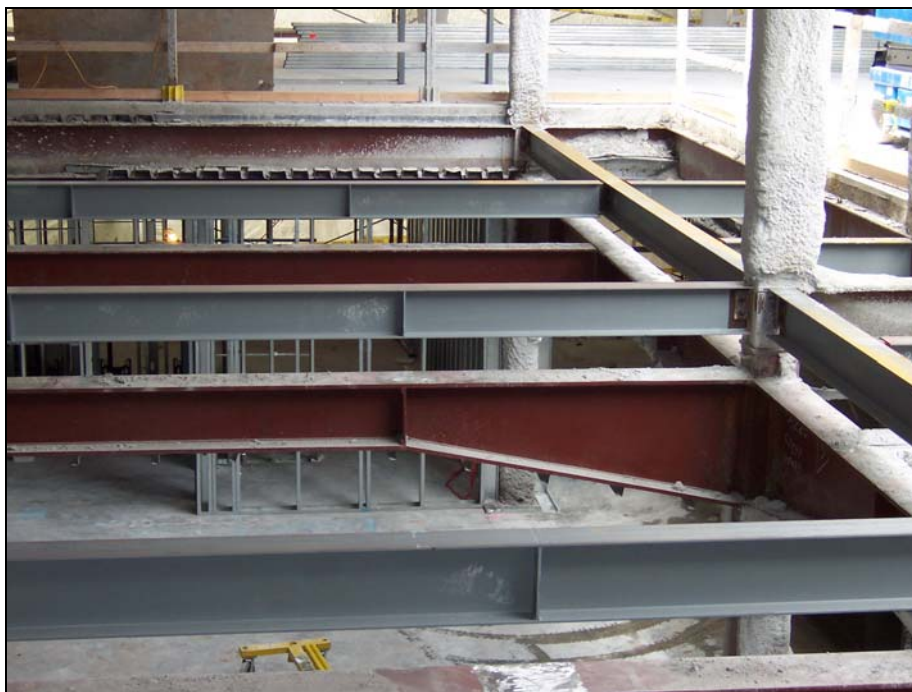
New Steel to Support New Deck at Second Floor
