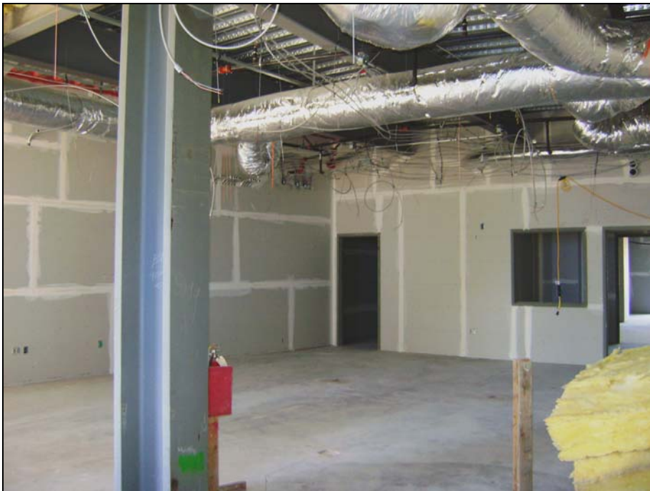
Interior MEP Rough-in and Drywall
