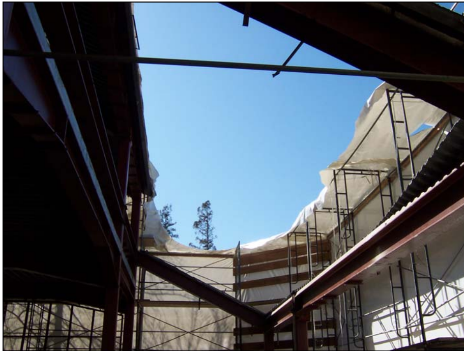
Northeast Portion of the Building Being Removed
