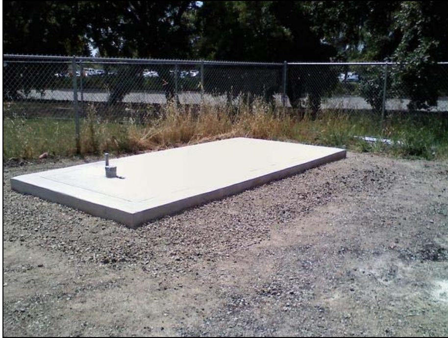
New Generator Pad
