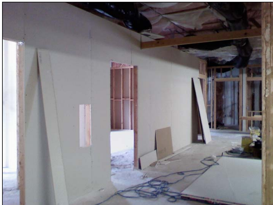
Installation of Gypsum Wallboard
