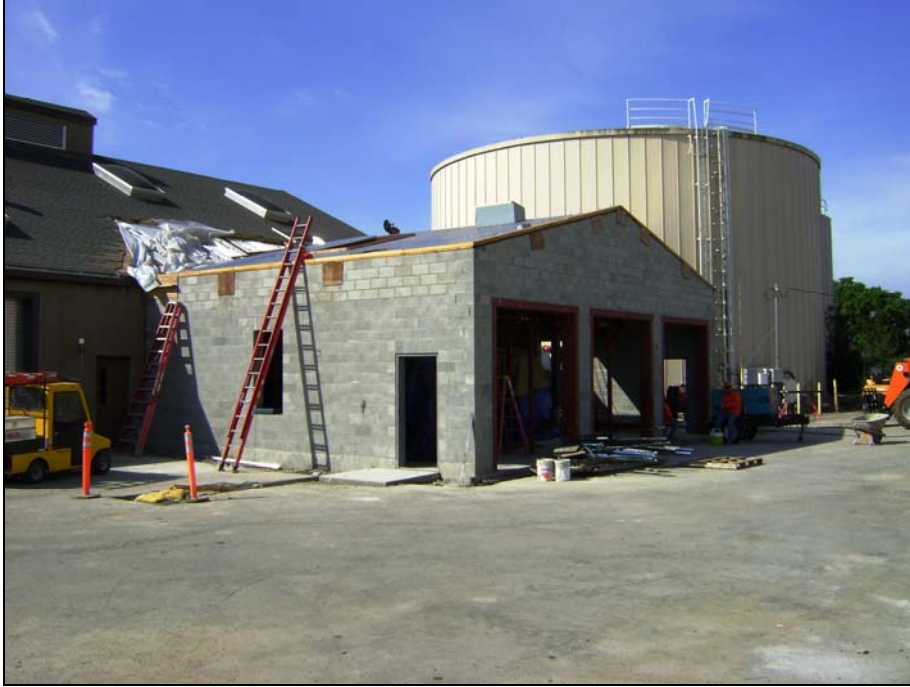
Chiller Building Addition
