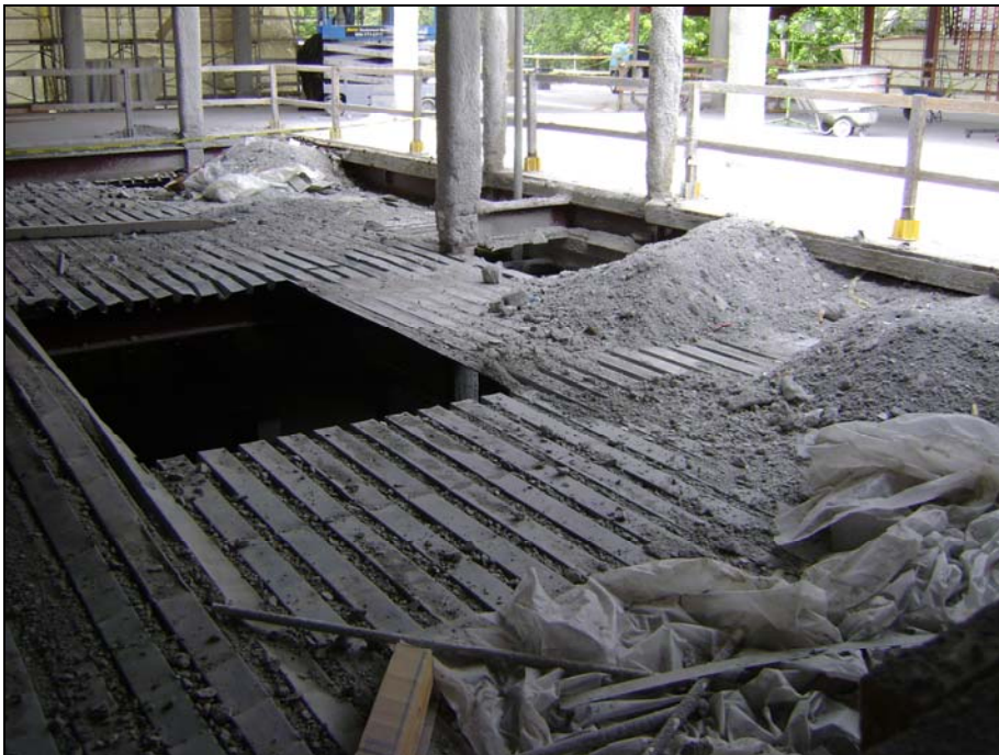
Demolition at Second Floor Depressed Deck
