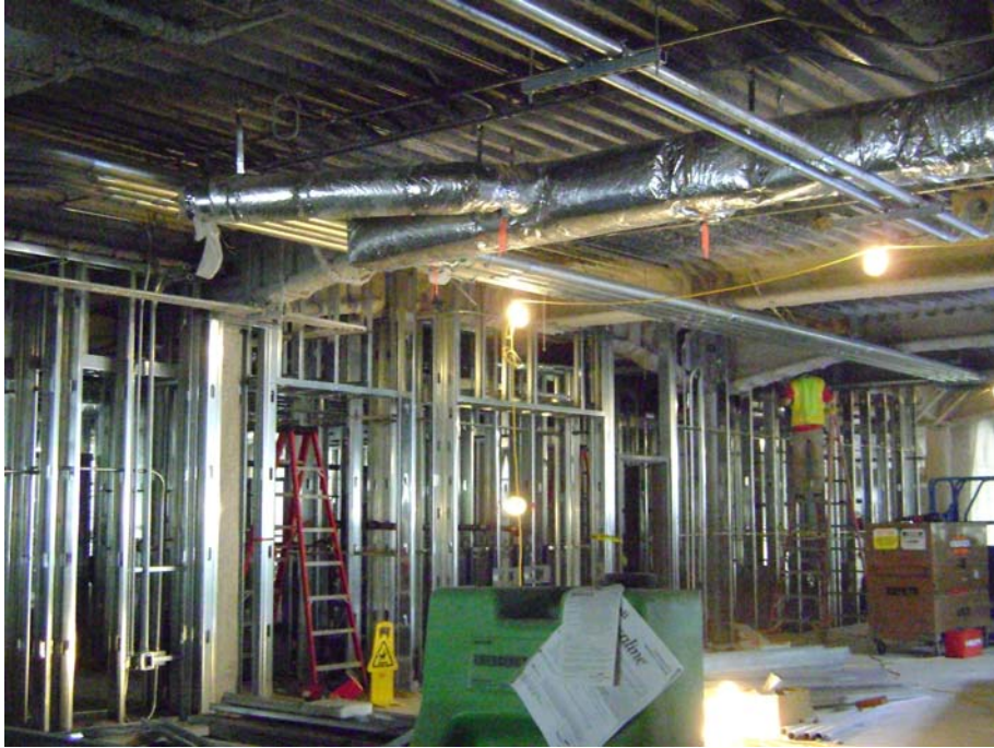
First Floor Framing, Plumbing, Mechanical & Electrical Well Underway
