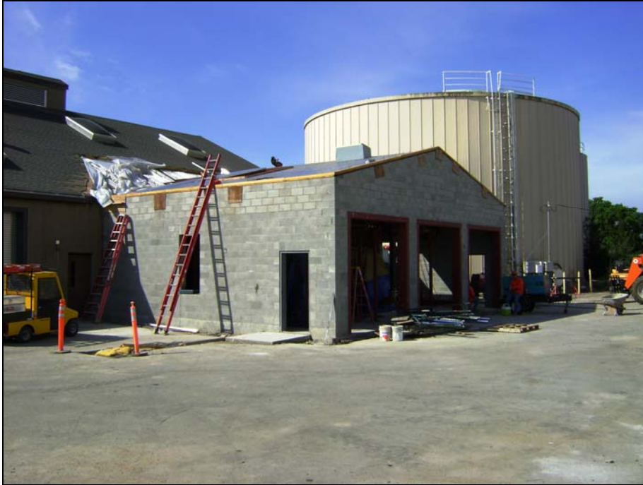
Chiller Building Addition
