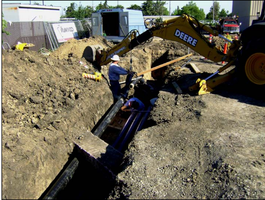
Hydronic Piping Installation
