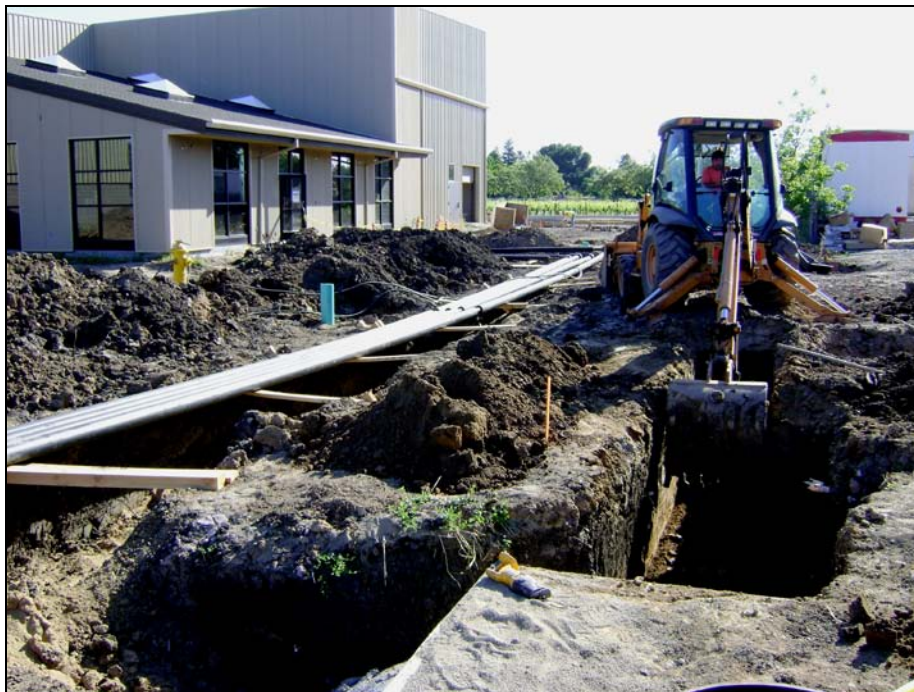
Generator Yard Excavation
