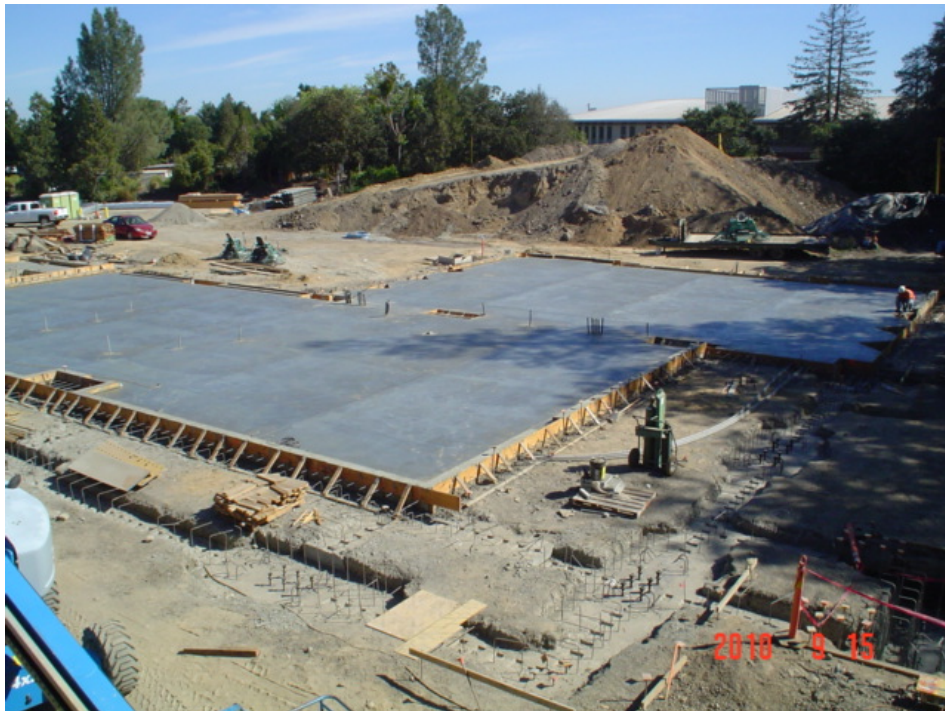
Placement of Concrete for Building Wing C
