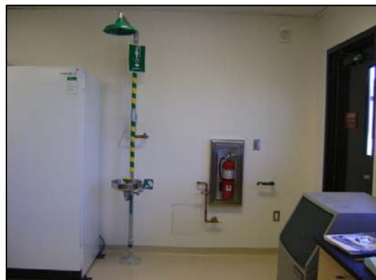
Portable 403 front, emergency shower
