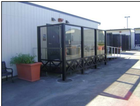
Restroom Portable 203 Windbreak
