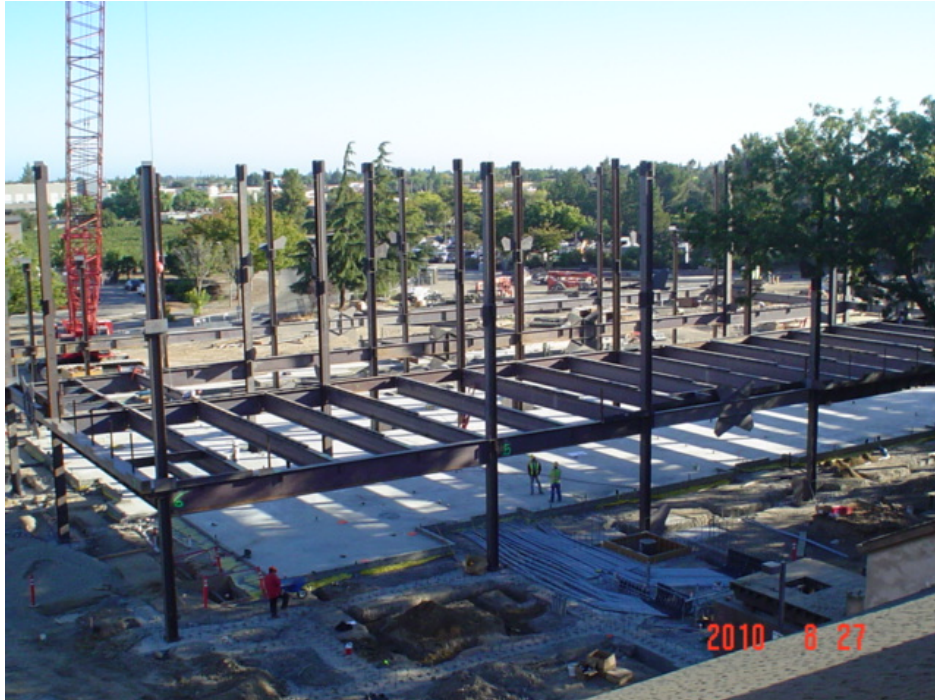
Building Wing A Structural Steel Installation
