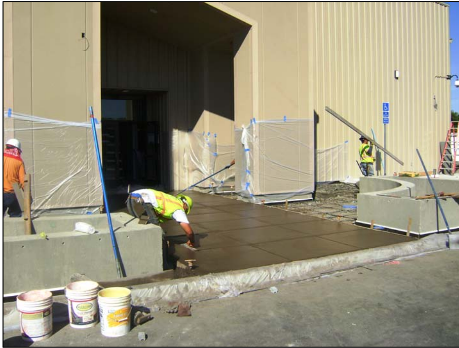
Entrance Raised Planters and Colored Concrete Placement
