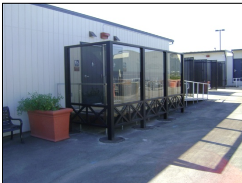
Restroom Portable 203 Windbreak
