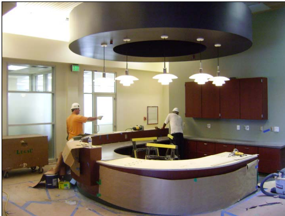
Customer Services Area – Casework Installation
