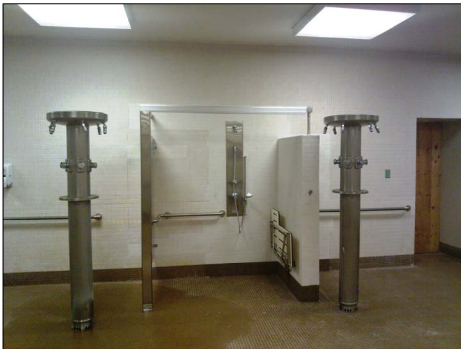
Men's Locker Room – Accessible Shower Stall
